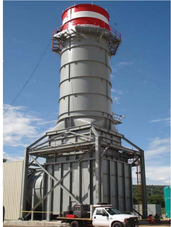
Convertible simple cycle exhaust stack for GE 7FA in Venezuela
