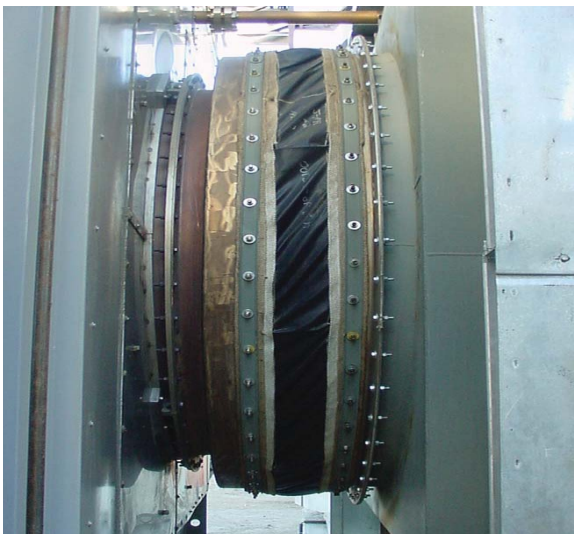
2260 mm (89") diameter Gas Turbine Exhaust Expansion Joint with Hot to Cold Frame. 25 in wc at 527°C (980°F)
